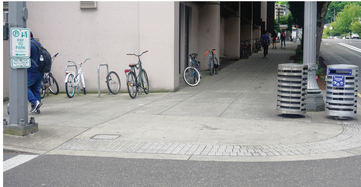
Above: Flush curb Right: Mountable curb detail
