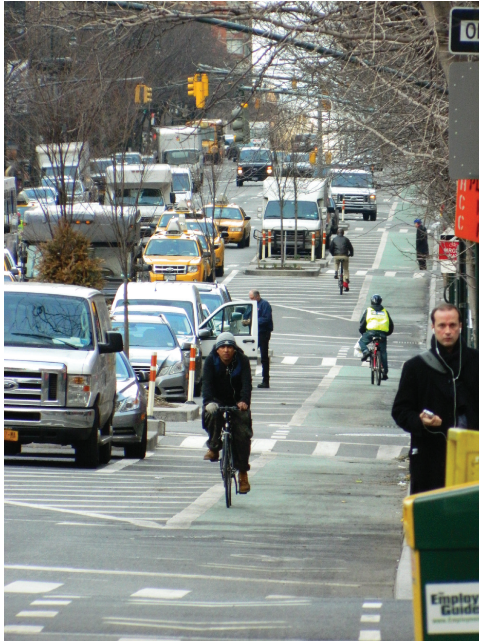
Wide bike lane installed on avenue in Manhattan
