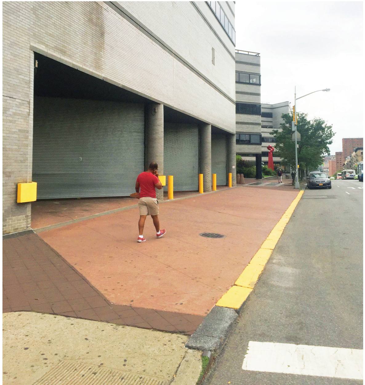
Painted sidewalk at loading dock entrance
